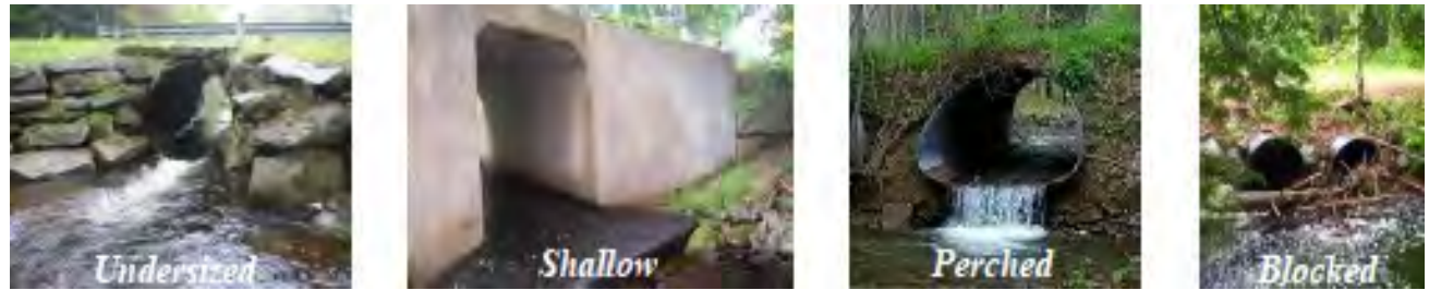
Barriers to fish passage include undersized, shallow, perched, and blocked culverts and bridge openings
